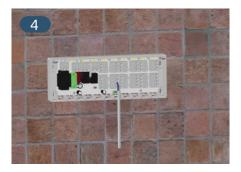
Lay the cables into the casing through the strain relief and install all cables to the basis using the clamping/plug-in technology; this is possible in a very short time.
